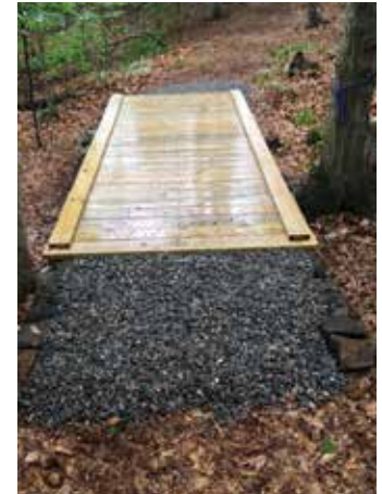
(Left photo) Bridge built over stream bed connecting trails in Chapman Mill Pond Open Space. (Right photo) Bridge frame with stone cribs on each end. Chapman Mill Pond Open Space. Photos by Tom ODell.
