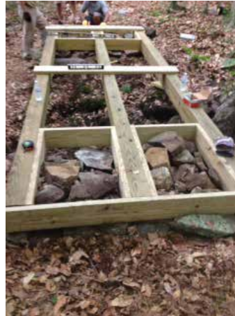
(Left photo) Bridge built over stream bed connecting trails in Chapman Mill Pond Open Space. (Right photo) Bridge frame with stone cribs on each end. Chapman Mill Pond Open Space. Photos by Tom ODell.
